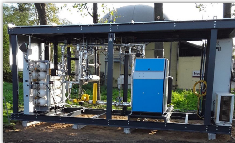
BioCNG-Hoftankstelle im Praxisbetrieb im Rahmen des RES4LIVE-Projekts. (Foto: ATB) BioCNG filling station in practical operation as part of the RES4LIVE project. (Photo: ATB)
