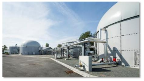
Main digester: 190 m<sup>3</sup> (165 m<sup>3</sup> reaction volume)
