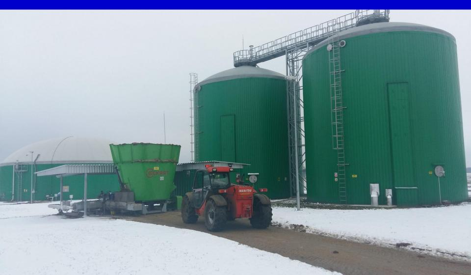
Study case – ProBioGas technology: agricultural-biowaste biogas plant in Miedzyrzec working with separated hydrolysis and long, narrow fermenters Agricultural-biowaste biogas plant (1200 kWe + 1300 kWt); 2 hydrolisys chambers (300 m<sup>3</sup> each), 2 fermenters (3300 m<sup>3</sup> each)
