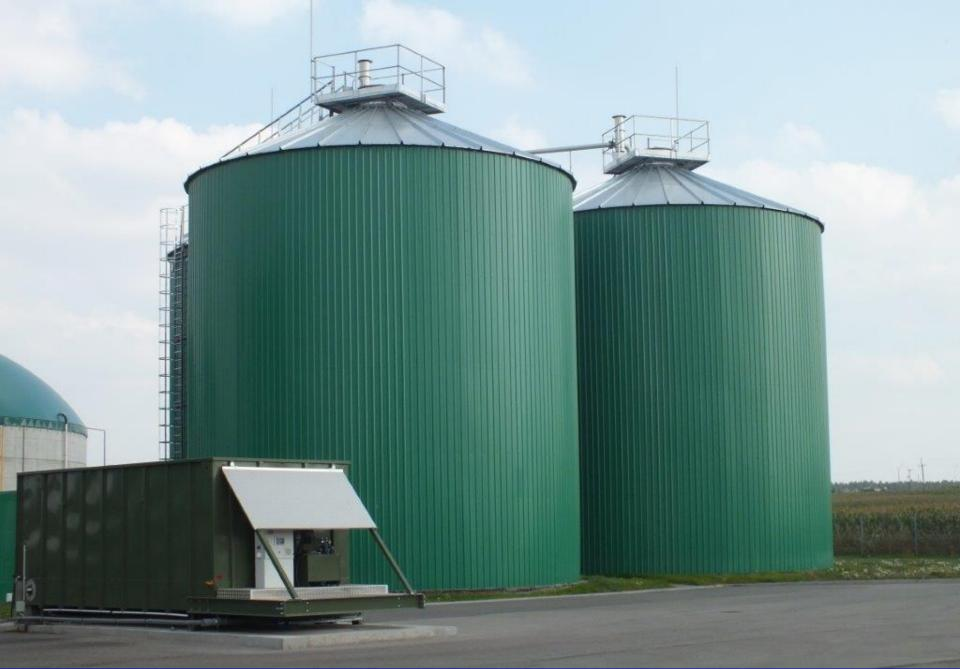
Extremely efficient mixing system (5 kW)  $\rightarrow$  very homogeneous pulp, no upper layer presence (even in case of maize silage with 44% D.M.)
